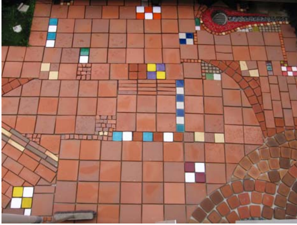
Courtyard under construction
