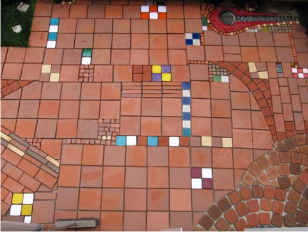
Courtyard under construction
